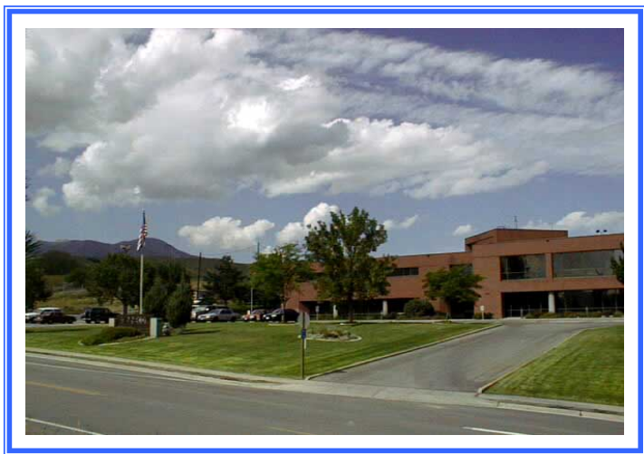
Kennecott’s Utah Copper’s corporate headquarters is located at the entry to the Historic Town Center.
